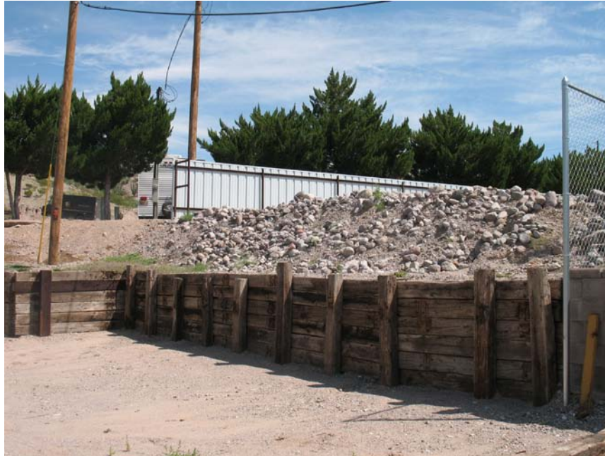
Grade stabilization on commercial site
